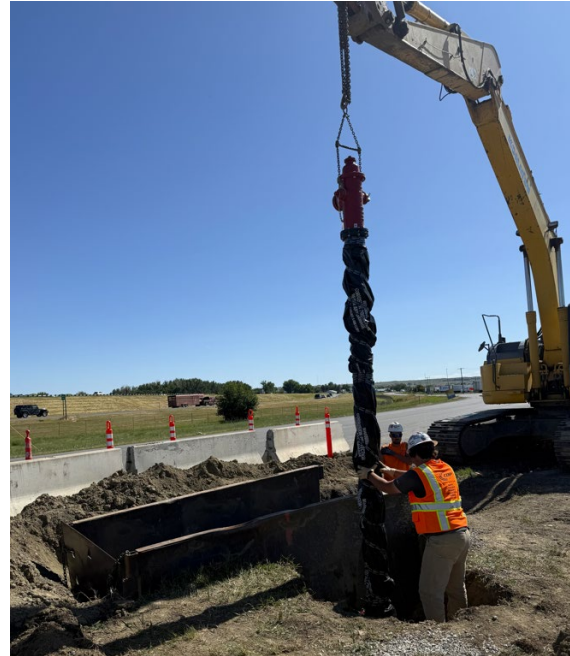
Left photo: 6/26/25, installation of the triple force main on the north end of the 42" interstate bore Right photo: 6/30/25, fire hydrant installation near the Town Pump
